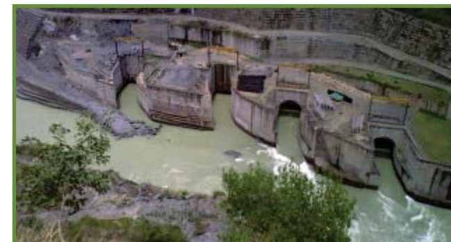
Diving Services on Koteswar Dam Project, Uttarakhand, India.
