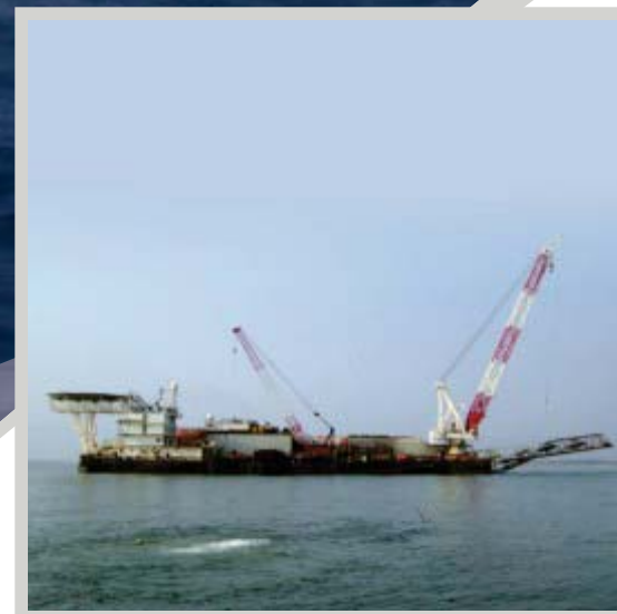
Diving support during Diffuser Installation for gas filed development project from Pipe lay barge 'Tug Mor', off Kakinada, A.P., India.
