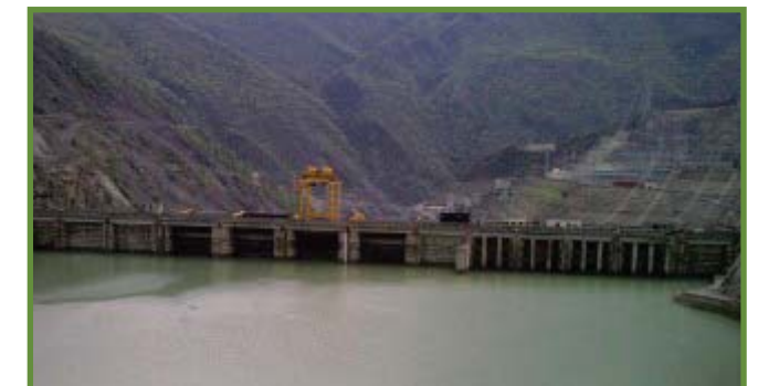
Diving Services on Tehi Dam Project, Uttarakhand, India.
