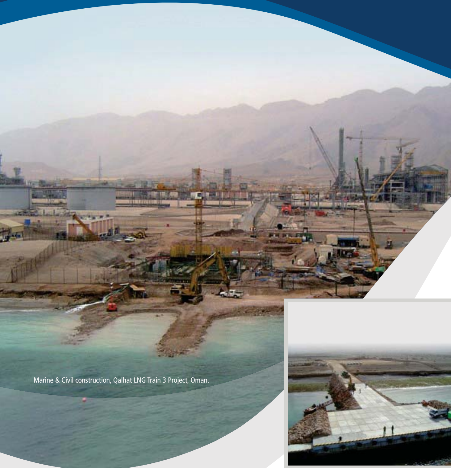
Temporary jetty constructed for loading, Qalhat LNG Train 3 Project, Oman.
