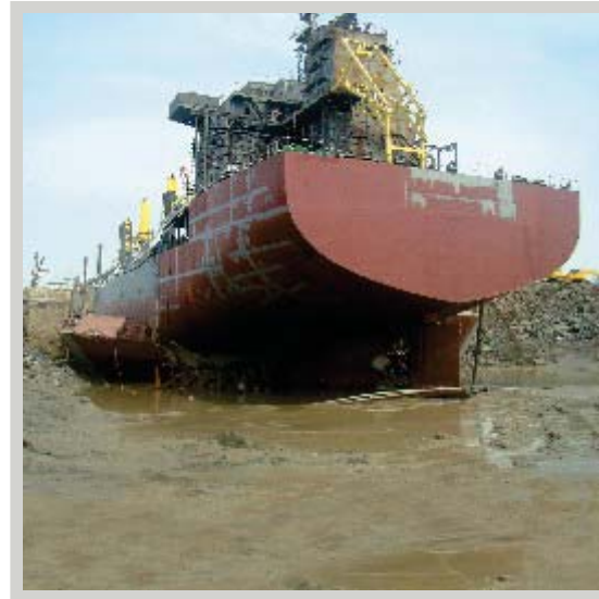
Ship damaged the shipyard's dry dock gates, Gujarat, India.
