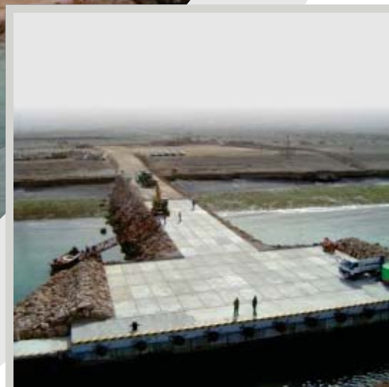
Temporary jetty constructed for loading, Qalhat LNG Train 3 Project, Oman.
