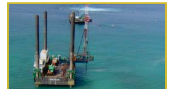
Spud barges on marine construction site, Muscat.
