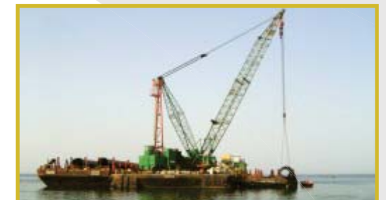
Intake Pipe laying, Altavela Power Project, Abu Dhabi.
